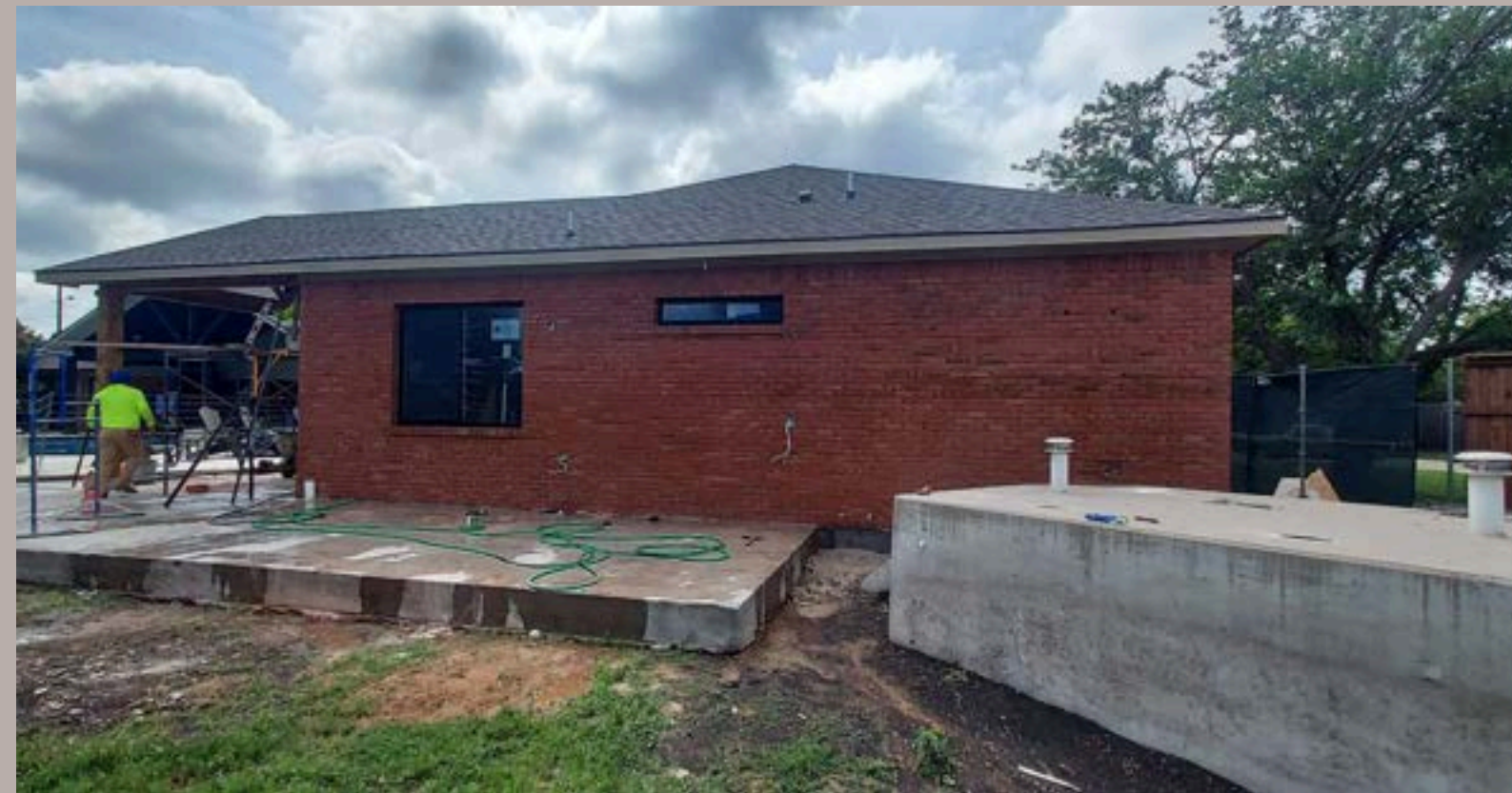
Celina TX 1600 sqft House built from ground up
